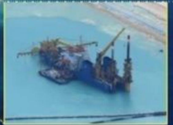
CUTTER SUCTION DREDGER
